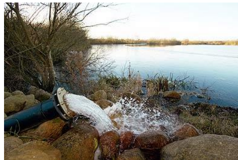
Figure 4: Artificial recharge outlet from Beder Water Works
